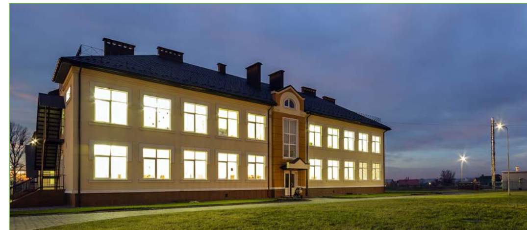
Use Ubiquity to manage school lighting schedules
