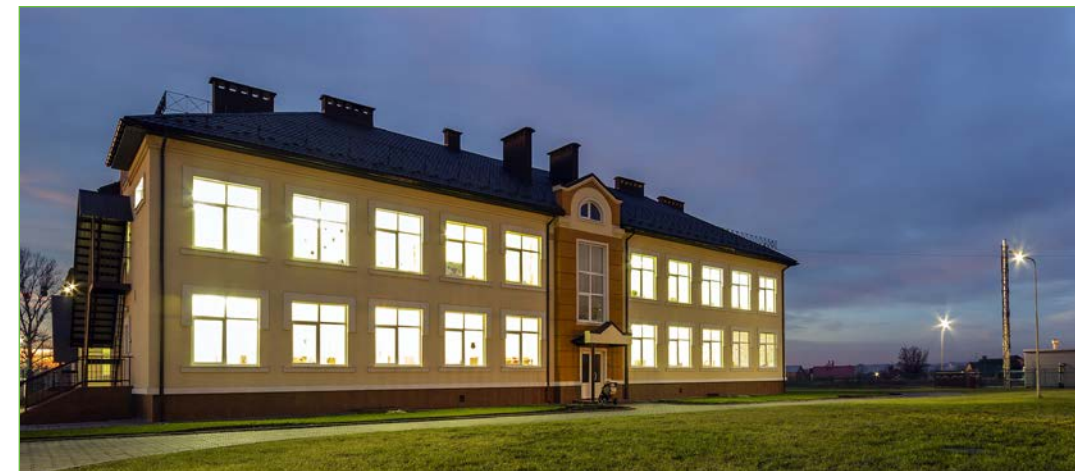
Use Ubiquity to manage school lighting schedules
