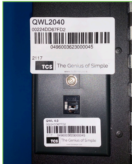
Placement of replacement Gateway label
