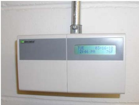
2. Place a simple thermometer (see note to the right) on top of the unit with the end that senses the temperature hanging over the edge. DO NOT USE A TEMPERATURE GUN. A temperature gun reads the surface temperature of whatever the gun is aimed toward, not the air temperature. And, we want to measure the air temperature.
