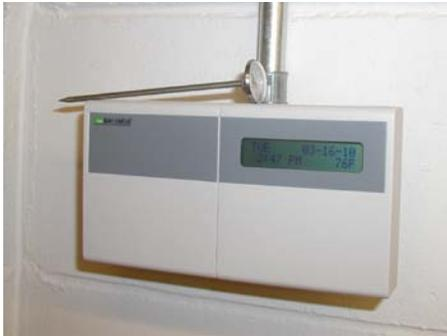
3. Modify the Calibration Offset value for the desired Temperature Input by adding or subtracting the required amount. This can be done on the programming page of the device within Ubiquity (see screenshot shown below) or using TCS Insight. Please reference Technical Support Bulletin 1019 for detailed instructions on using TCS Insight to calibrate sensor inputs.
