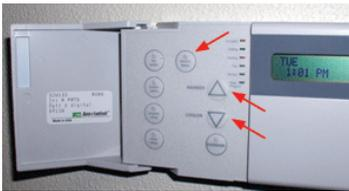
**Changing Setpoints:** To change the setpoints on the thermostat, simply flip open the cover and press either the “Warmer” or “Cooler” button. You will then see the Heat and Cool setpoints raise or lower on the display. These new setpoints will be used by the thermostat for programmed of hours or until changed again using the Warmer/Cooler buttons. Pressing the “Service Status” button will return to the Main Display showing the Time/Day/Date and current temperature.
