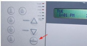
**After Hours Operation:** Pressing the "Override" button will change the thermostat from its unoccupied "Night Setback" setpoints to the occupied set points for a pre-programmed period, or until the Override button is pressed again.
