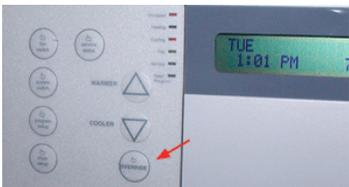
**After Hours Operation:** Pressing the “Override” button will change the thermostat from its unoccupied “Night Setback” setpoints to the occupied set points for a pre-programmed period, or until the Override button is pressed again.
