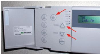
**Changing Setpoints:** To change the setpoints on the thermostat, simply flip open the cover and press either the "Warmer" or "Cooler" button. You will then see the Heat and Cool setpoints raise or lower on the display. These new setpoints will be used by the thermostat for programmed hours or until changed again using the Warmer/Cooler buttons. Pressing the "Service Status" button will return to the Main Display showing the Time/Day/Date and current temperature.
