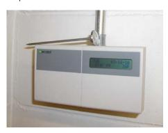
Modify the Calibration Offset value for the desired Temperature Input by adding or subtracting the required amount. This can be done on the programming page of the device within Ubiquity (see screenshot shown below) or using TCS Insight. Please reference Technical Support Bulletin 1019 for detailed instructions on using TCS Insight to calibrate sensor inputs.
